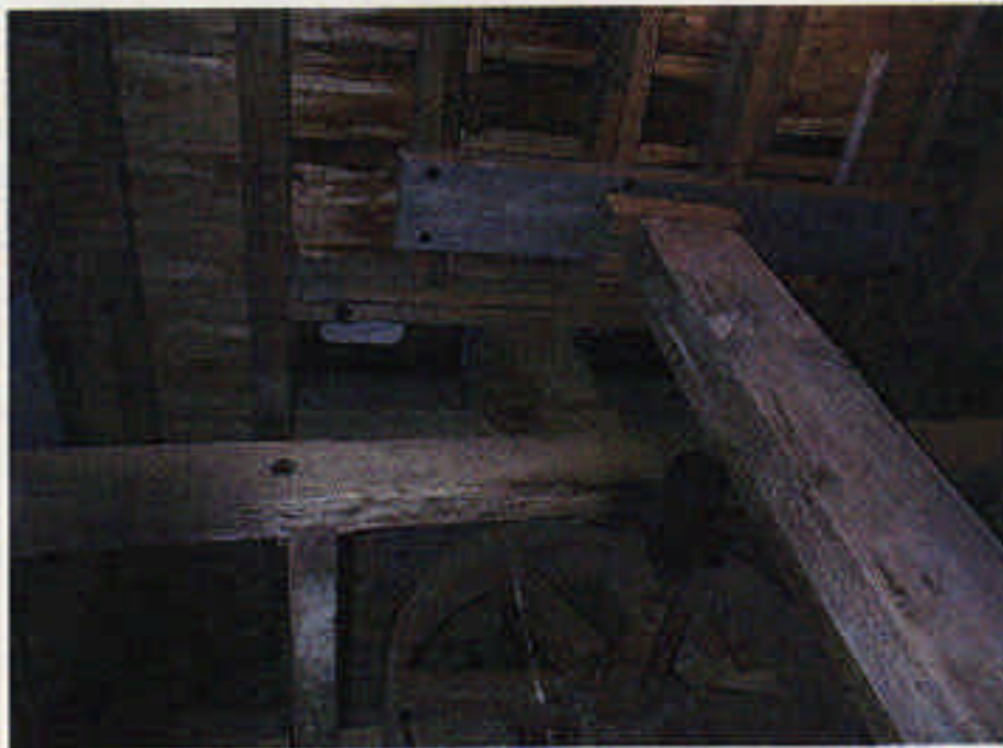
Photograph 6: New column near the hopper opening.
