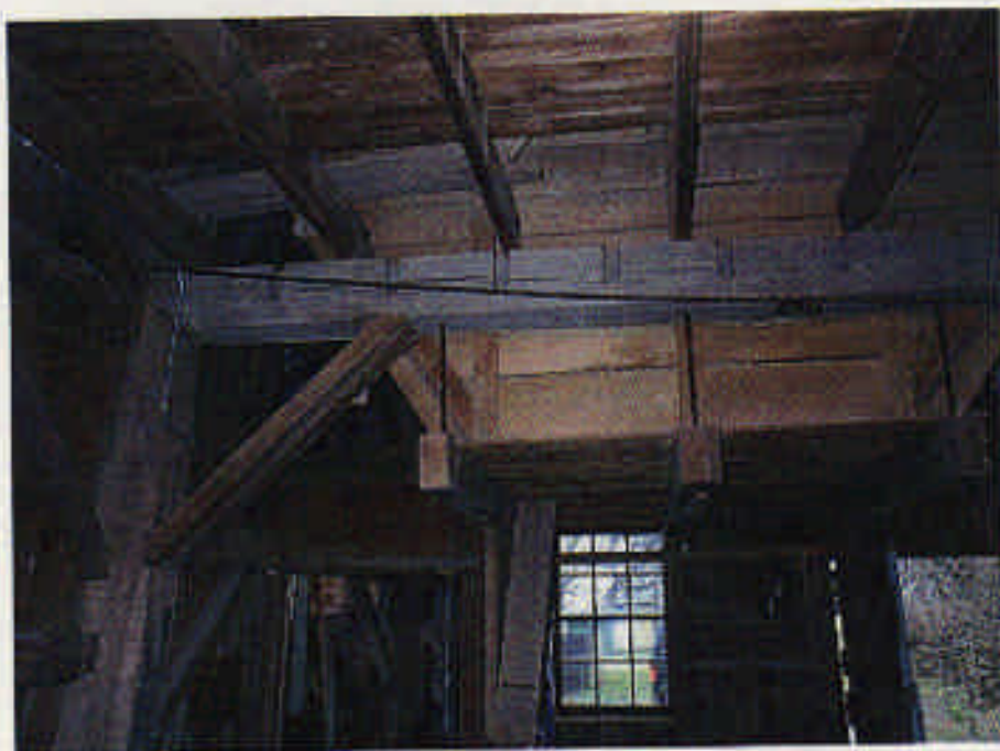
Photograph 2: Floor framing at mezzanine level.
