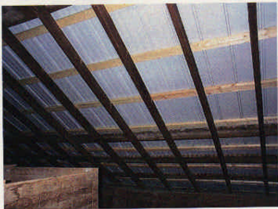
Photograph 1: Roof purlins, rafters and metal deck
